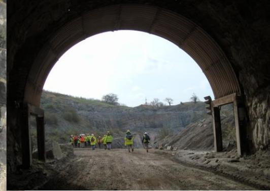
The tunnel connects the two quarries at Tytherington, passing through the Gully Oolite Formation.
